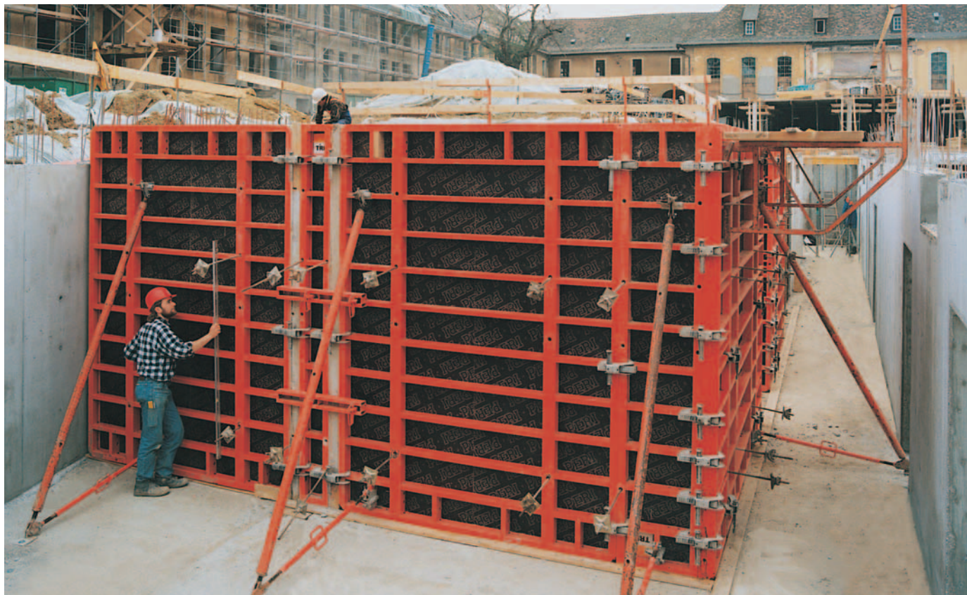
The BFD alignment coupler
